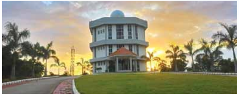
X-band radar building at NARL
