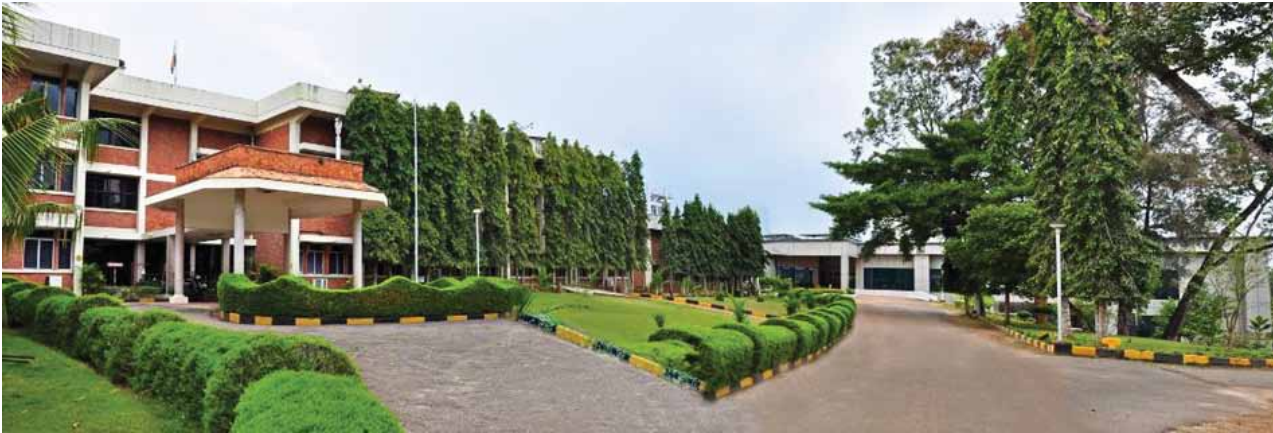
IISU Main Building
