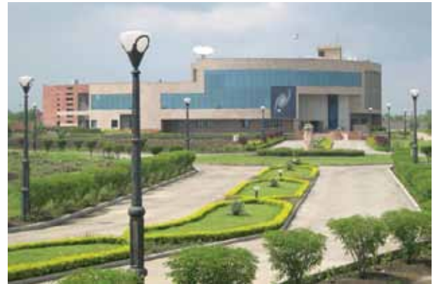
Satellite Control Centre – MCF, Bhopal
